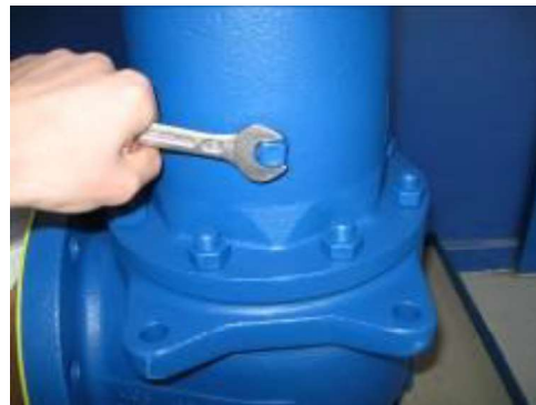
Fig. 2 Sealing the drain hole
